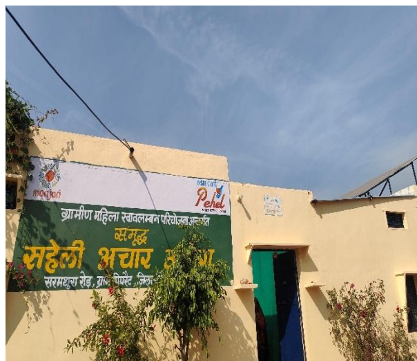
Image 22: Pickle Unit Pipret with solar panels
