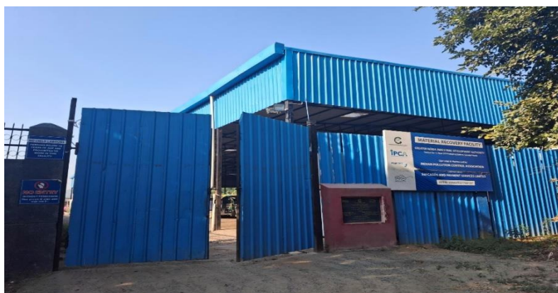
Figure 11: Material recovery facility, Greater Noida
